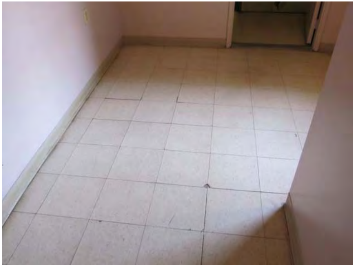
Worn/loose vinyl tiles noted at some common hallway floors
