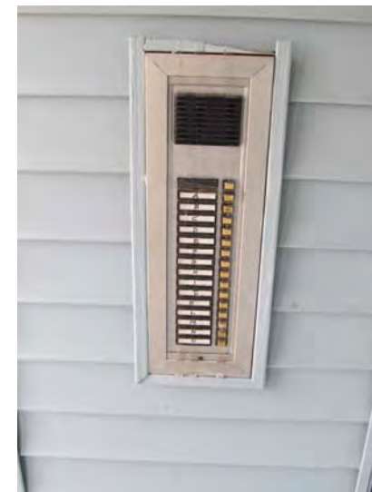
Typical original door buzzer/intercom panel found at each of the building's four common entries
