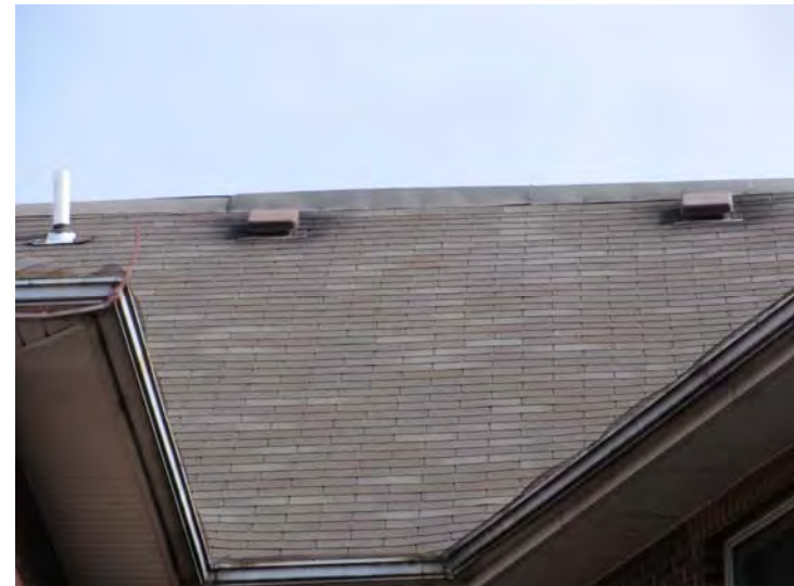
Original roof shingles are at or near the end of their expected useful service life and exhibit age-related wear
