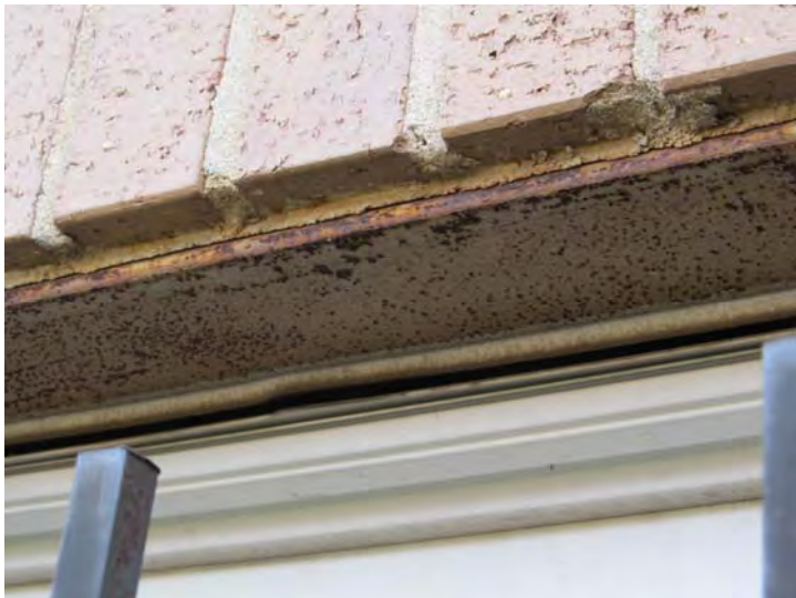
Steel lintels at window openings are in need of surface preparation and painting
