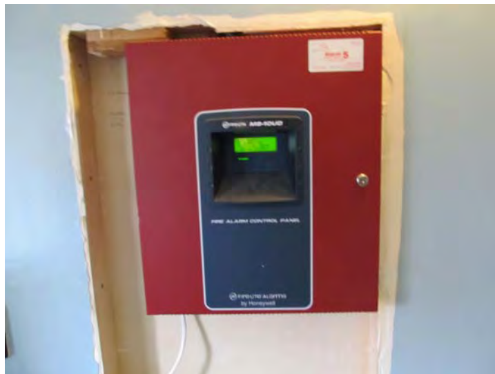
Typical newer, fully addressable, fire alarm control panel found at each of the building's two street addresses
