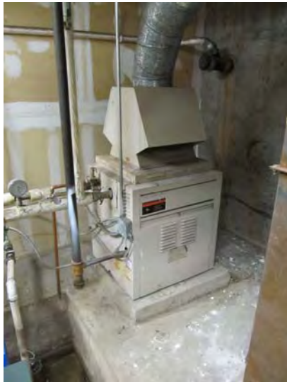
Original boiler for generation of domestic hot water
