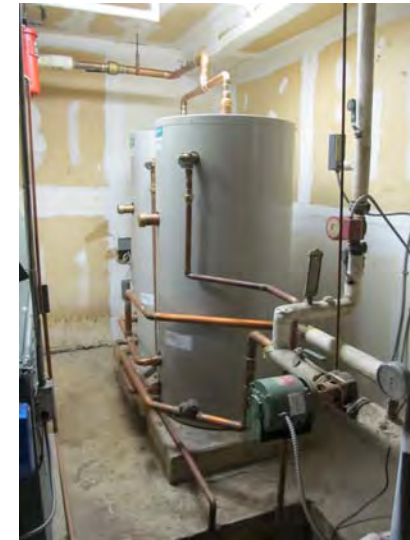
Domestic hot water storage tanks – New anode rods recently installed
