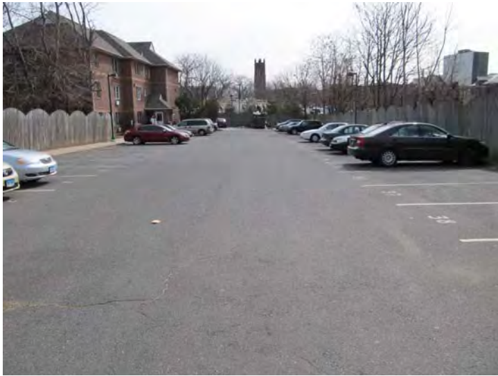
Asphalt paving is in generally good condition – Routine surface maintenance needed in near-term
