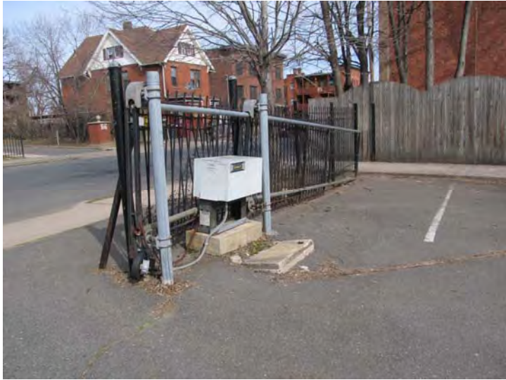
Motorized operator for gate at entry to parking area is currently offline
