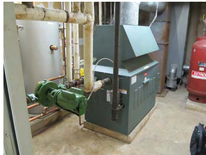
Recently installed boiler and pump for generation and distribution of hydronic heat throughout the building
